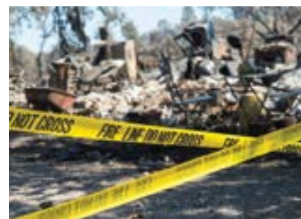
The sooty remains of a home destroyed by last year's Middletown fire show the sad consequence of roaring wildfires. Middletown is rebuilding and will be better than ever with help.
